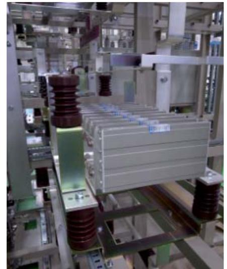
Figure 6: Fuses with low inductance for IGBT protection
